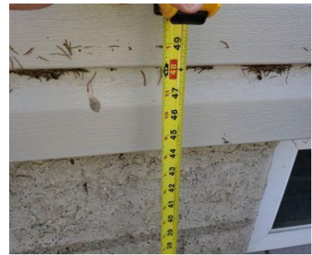
Debris Deposits in Waterways Area
